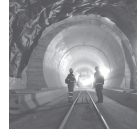
The Gotthard Base Tunnel while under construction
